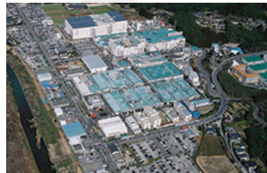
Sendai Facility (JAPAN)
