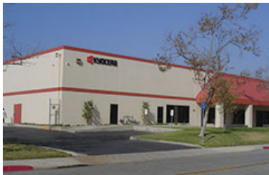
California Facility (USA)
