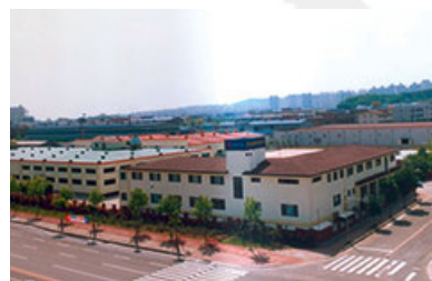
Incheon Facility (KOREA)
