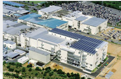
Yokaichi Facility (JAPAN)
