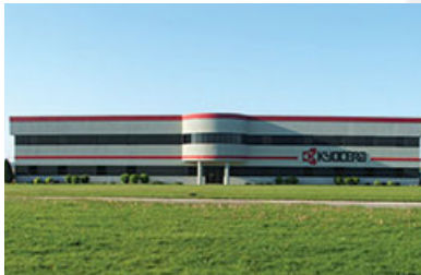
Ohio Facility (USA)
